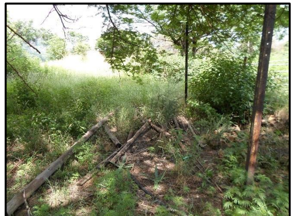
Figure 8-7. Broken down structure (Point 3)
