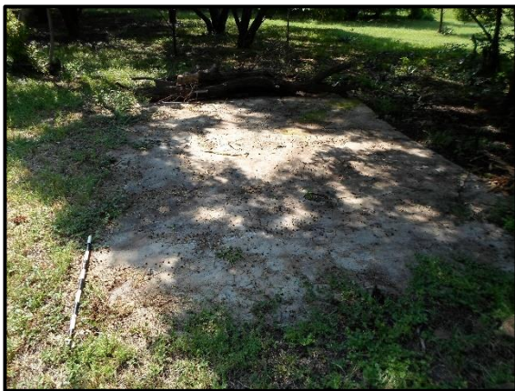
Figure 8-6. Cement foundations of a structure (Point 2).
