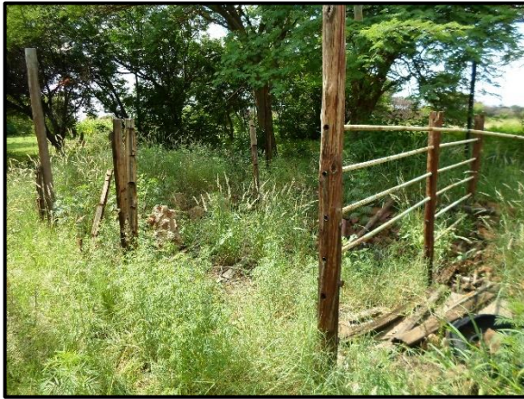
Figure 8-8. Remains of structure at Point 3.
