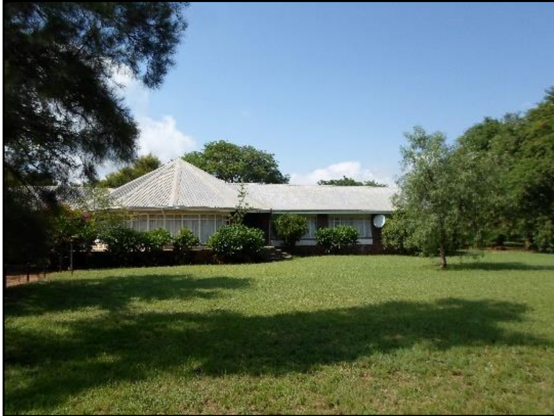
Figure 5-1. General site conditions at the main dwelling.
