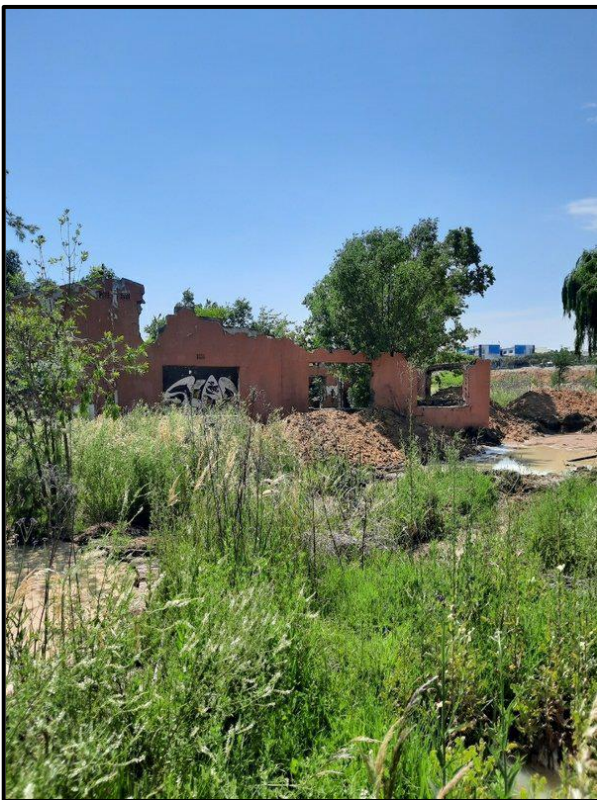
Figure 8.4. Dilapidated structure at Waypoint 235.
