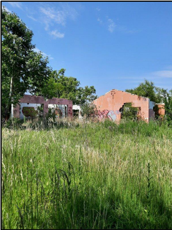
Figure 8.2. Demolished structure at Waypoint 235
