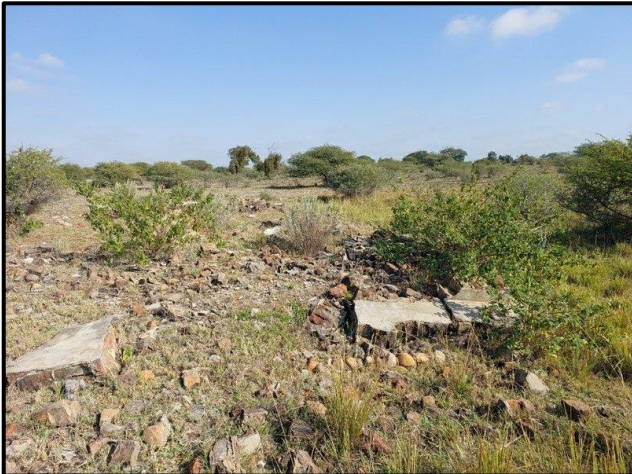
Figure 8.12. Building rubble present at K002.
