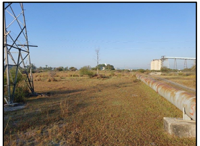
Figure 7.4. General site conditions.
