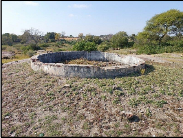
Figure 8.10. Water reservoir no longer in use at K002.
