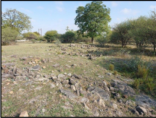
Figure 8.2. Series of broken-down foundations at K001.
