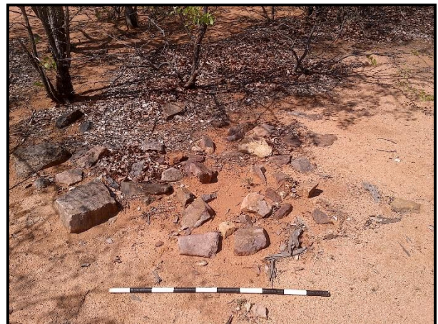
Figure 32. Grain bin foundations
