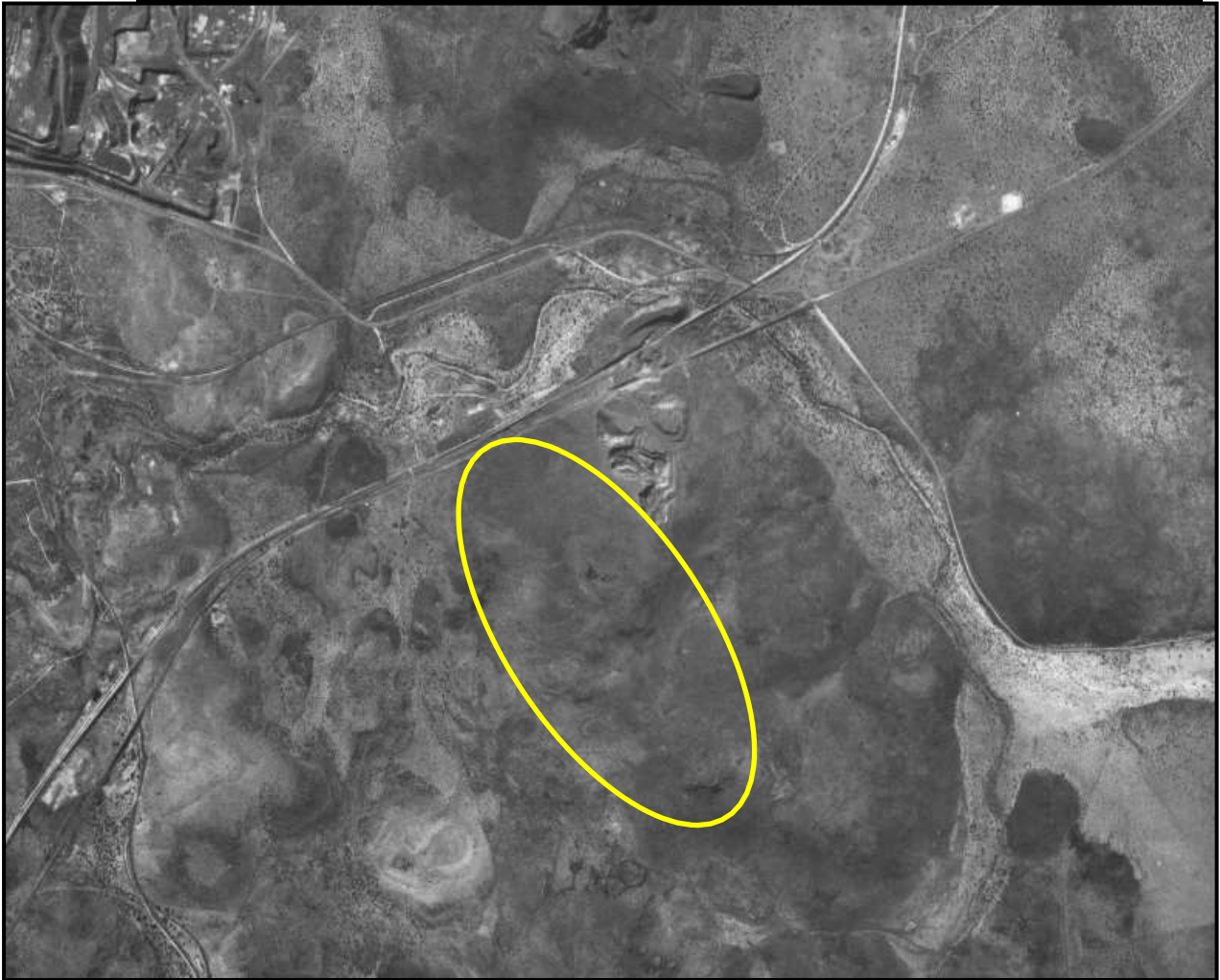
Figure 7: 1988 Aerial Image of the Study Area. By This Time the N14 was Built with Limited Mining Activity in the Surrounding Area
