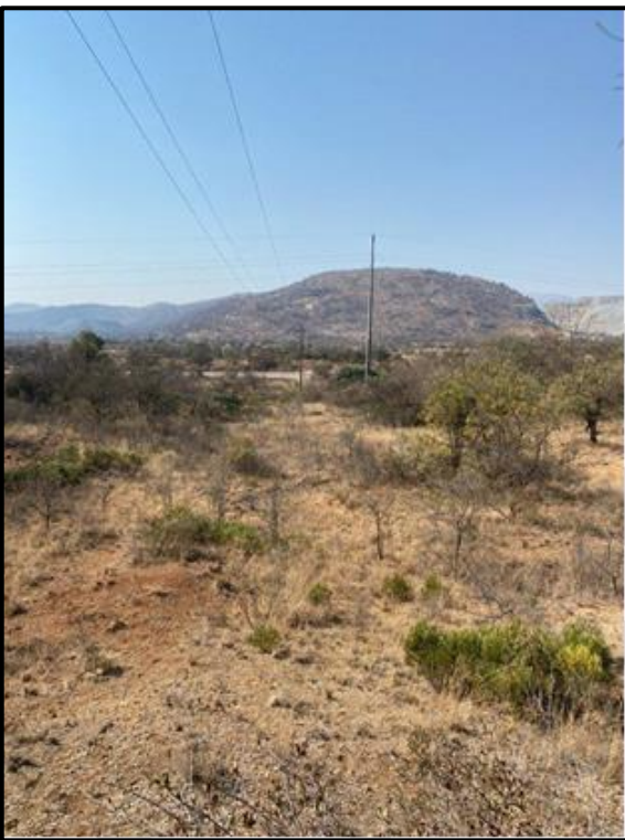
Figure 7.3. Powerline in the RWD area.
