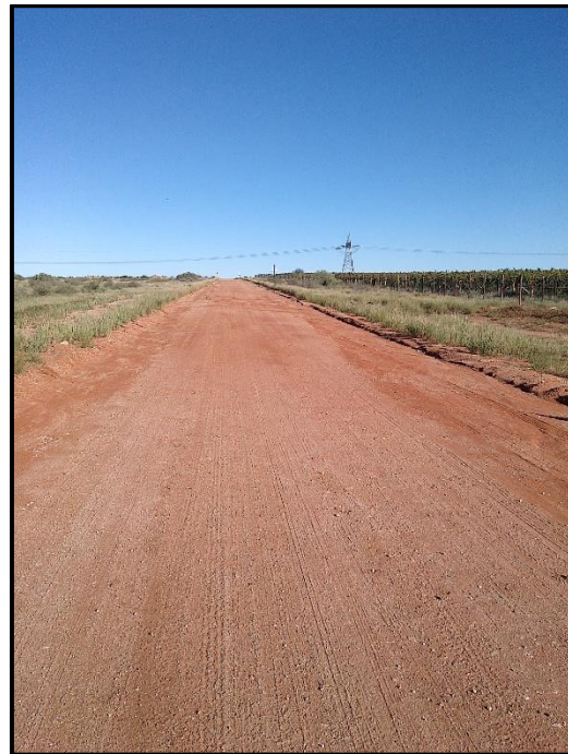
Figure 7.4. Existing access road to the study area.
