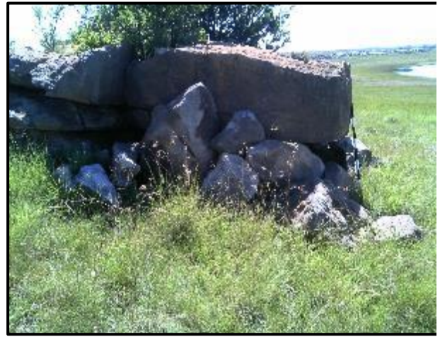
Figure 41. Dry stone wall.
