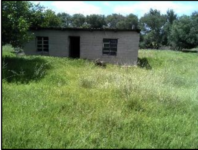
Figure 27. Abandoned dwelling at KP13.
