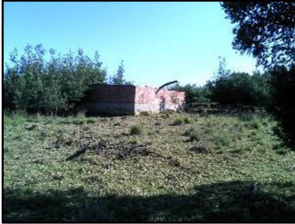
Figure 23. Structure at KP 11.
