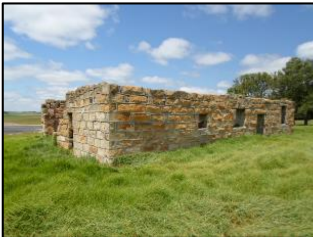
Figure 38. Structure at KP 22.
