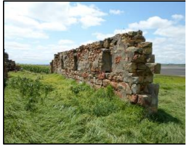
Figure 37. Wall at KP 22.
