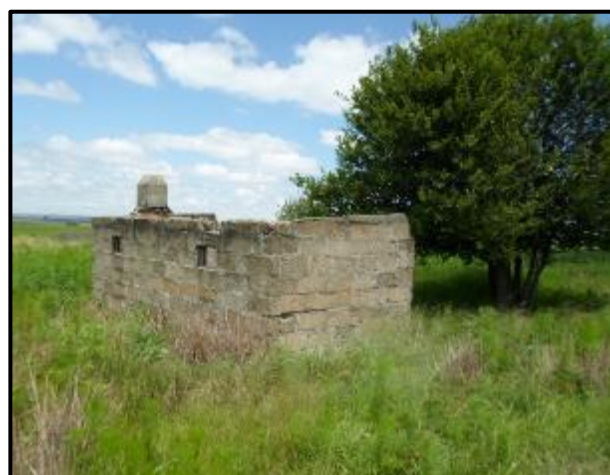
Figure 18. Structure at KP 6.
