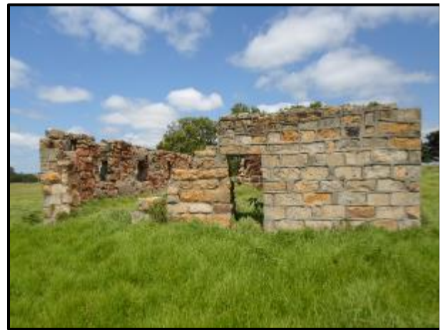
Figure 39. Structure at KP 22.
