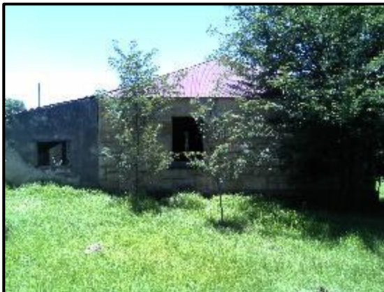
Figure 21. All the fittings have been removed.
