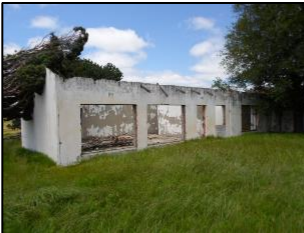
Figure 34. Structures at KP 21.
