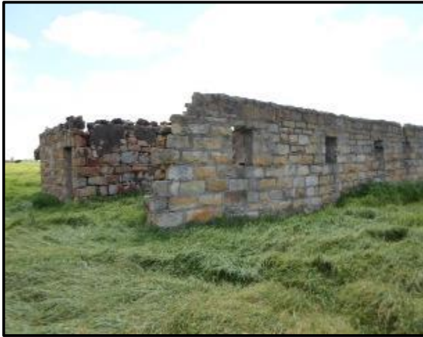
Figure 36. Structure at KP 22.
