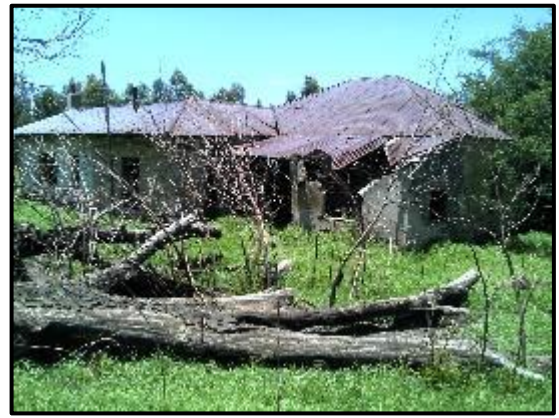
Figure 22. General site conditions.
