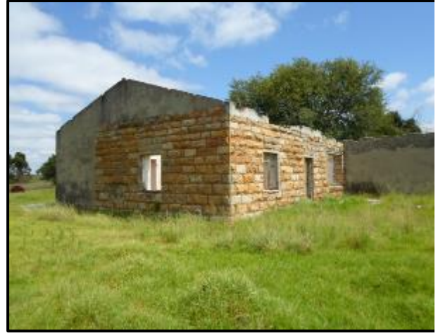
Figure 33. Structures at KP 21.
