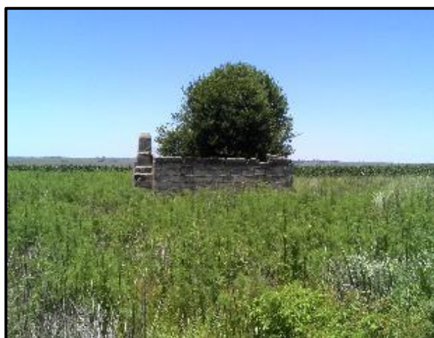
Figure 17. Structure at KP6.
