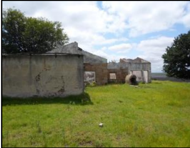
Figure 32. Structures at KP 21.
