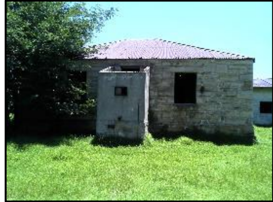
Figure 20. Structure with hipped roof.
