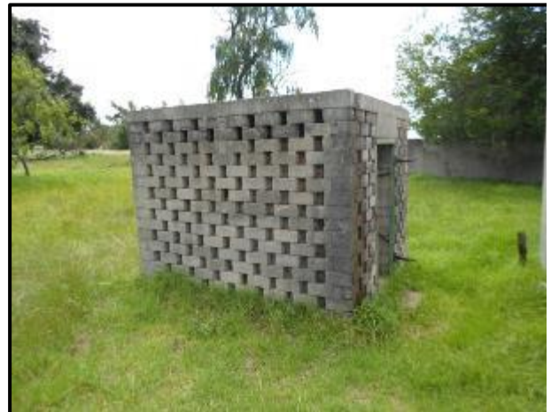
Figure 35. Structures at KP 21.
