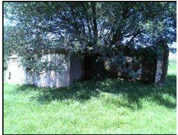
Figure 29. General site conditions at KP 15.
