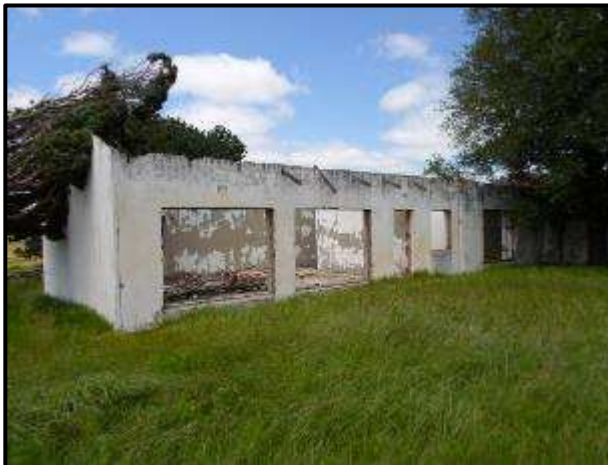
Figure 34. Structures at KP 21.
