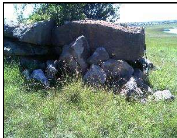
Figure 41. Dry stone wall.
