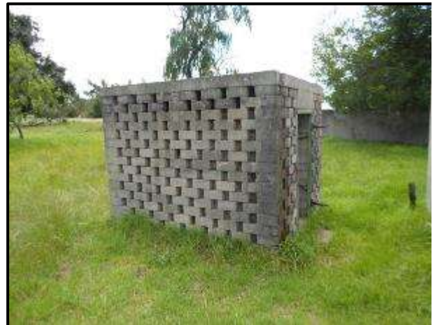
Figure 35. Structures at KP 21.
