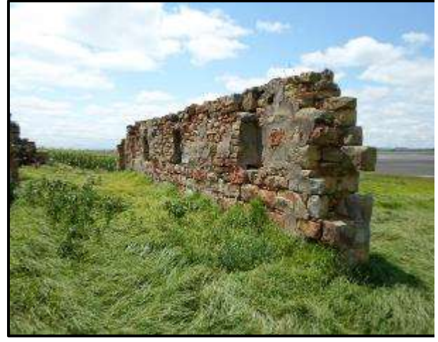
Figure 37. Wall at KP 22.
