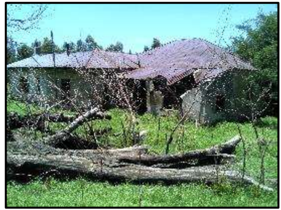
Figure 22. General site conditions.
