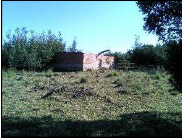
Figure 23. Structure at KP 11.
