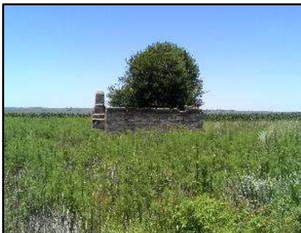
Figure 17. Structure at KP6.
