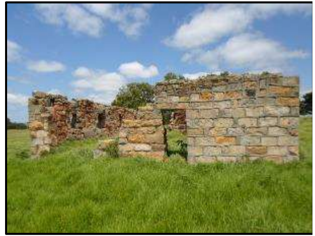
Figure 39. Structure at KP 22.
