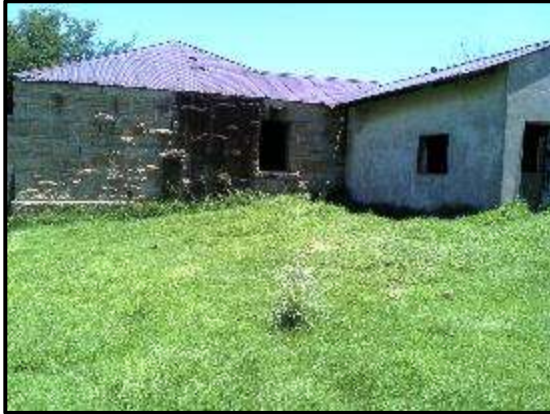
Figure 19. Structure with added on plastered sections.
