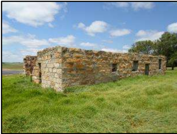
Figure 38. Structure at KP 22.
