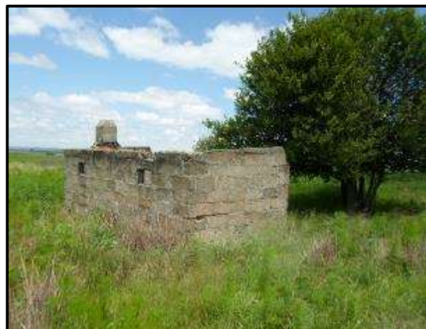
Figure 18. Structure at KP 6.
