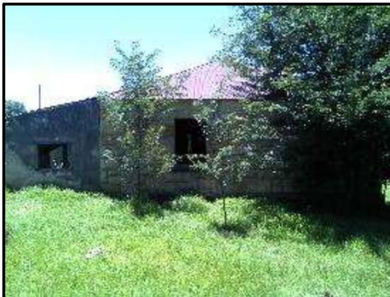
Figure 21. All the fittings have been removed.
