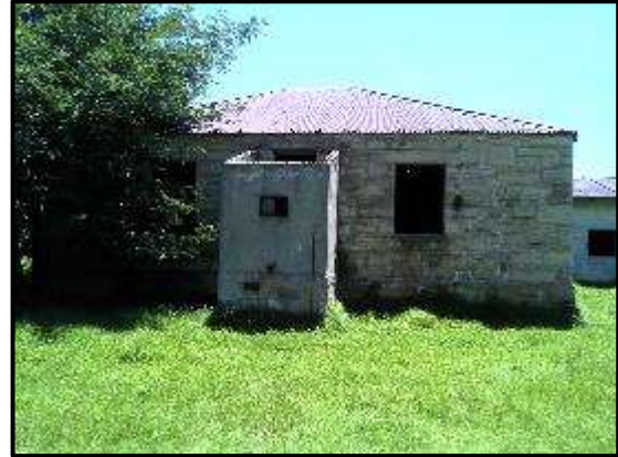
Figure 20. Structure with hipped roof.
