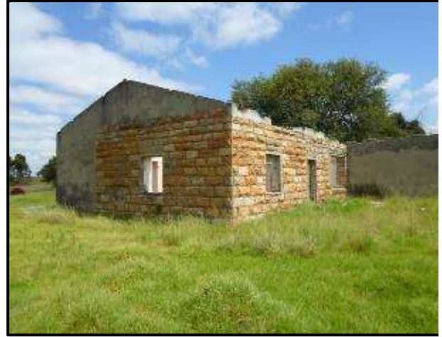
Figure 33. Structures at KP 21.
