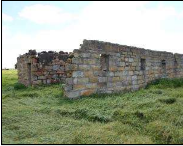
Figure 36. Structure at KP 22.
