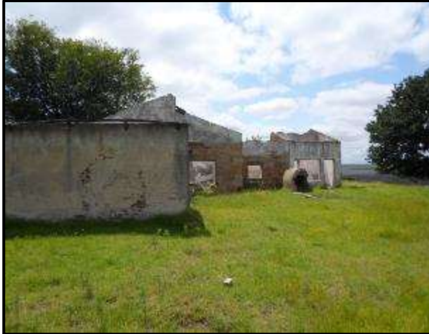
Figure 32. Structures at KP 21.
