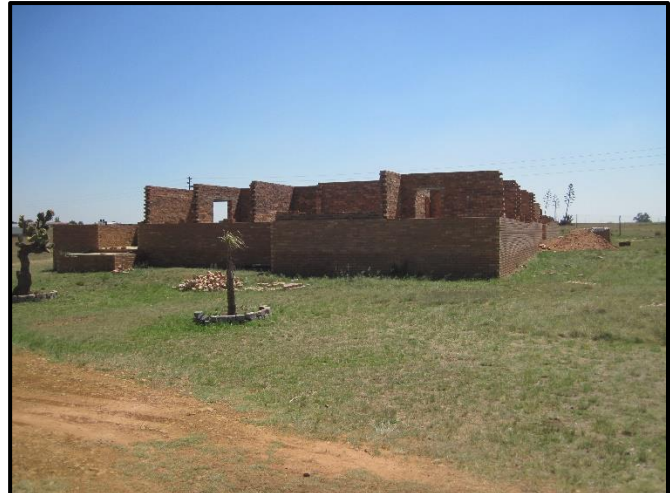
Figure 9. General site conditions – existing structures.
