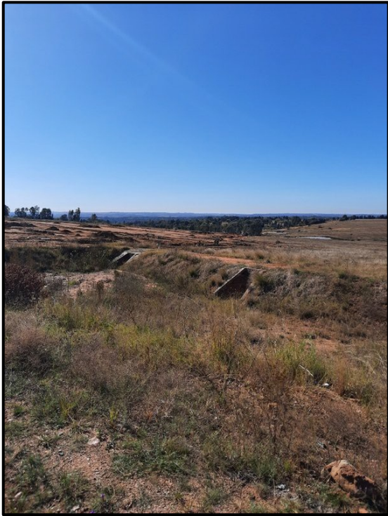
Figure 7.1. General site conditions – Large scale construction works towards the northern edges of the project area.
