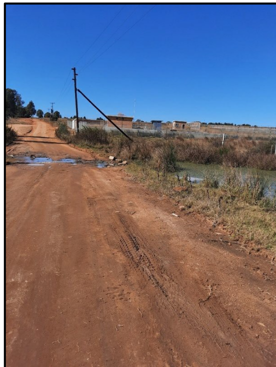
Figure 7.4. General site conditions – Small water treatment plant on the north-eastern edge of the project area.
