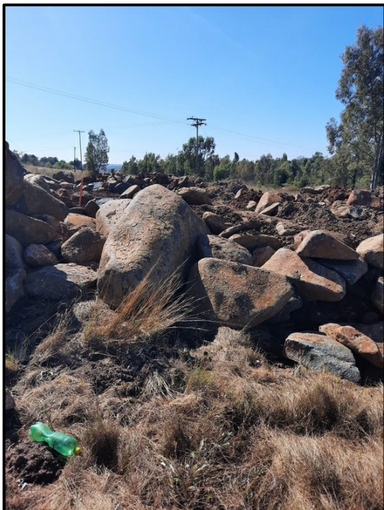
Figure 7.3. Current construction activities spilling over into the proposed project area.
