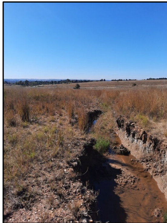
Figure 7.8. Erosion taking place along the drainage line into the wetland area.
