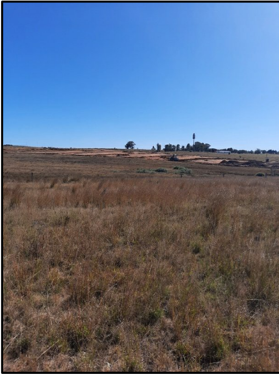
Figure 7.5 General site conditions -dense grass cover throughout the southern half of the proposed project area.
