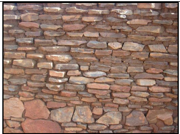
Figure 38. Construction technique at Site 15
