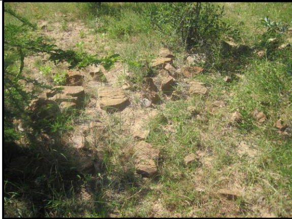
Figure 33. General site conditions Site 8
