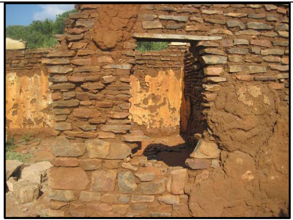
Figure 36. Stone lintel in window
