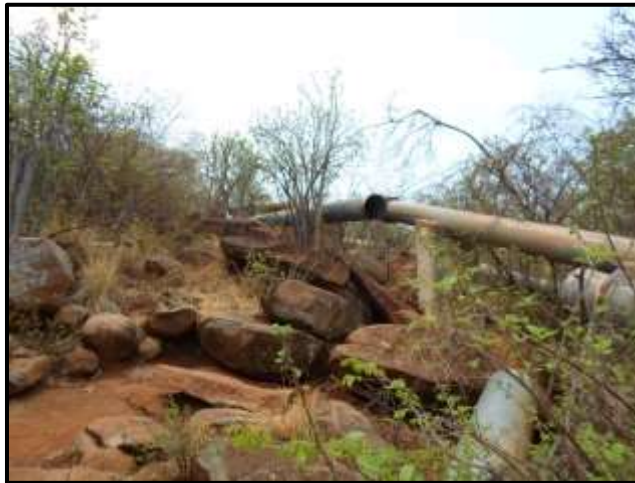
Figure 25. Old existing pipeline
