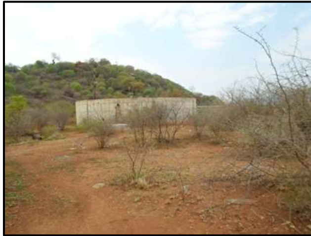
Figure 24. Cleared area around water reservoir
