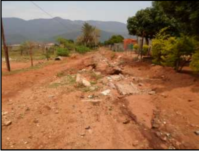
Figure 7. General site conditions.
