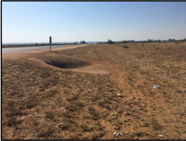
Figure 8. Witfontein Borrow Pit 3 – General site conditions
