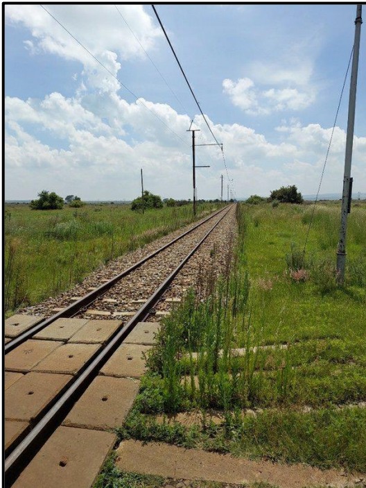
Figure 7.3. Existing railway in the study area.
