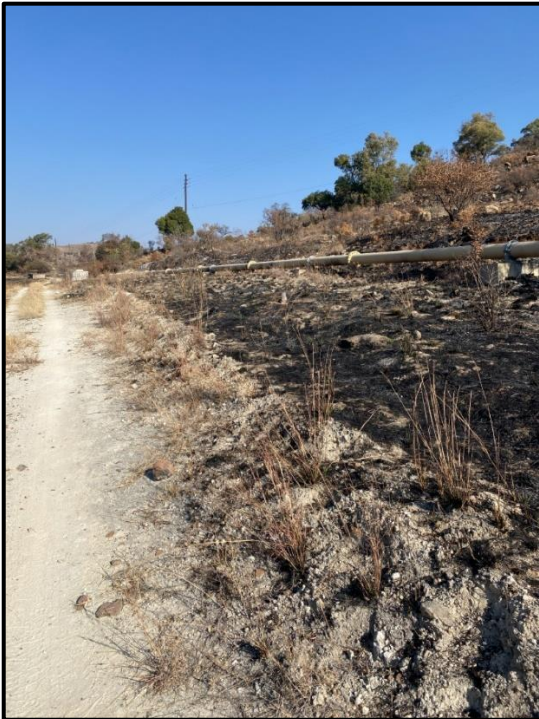
Figure 7.3. Existing pipeline in the servitude.
