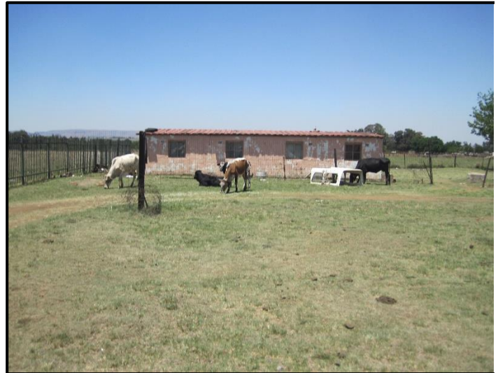
Figure 9. General site conditions – existing structures.
