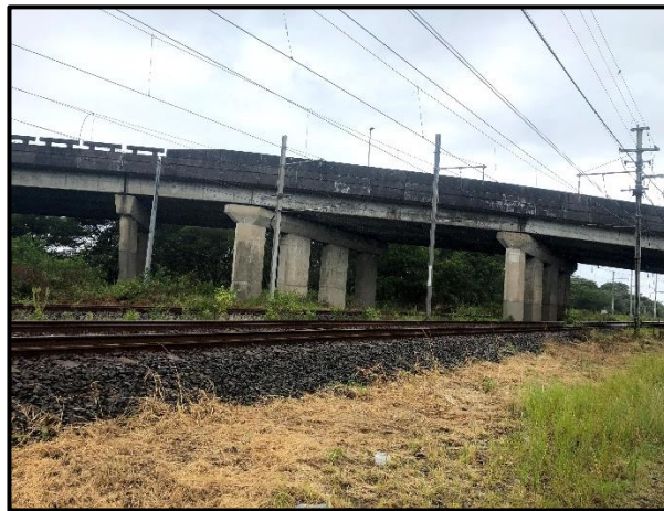
Figure 5-3. Railway lines and roads in the Port area.
