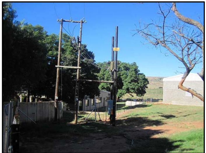
Figure 7. Existing transformer
