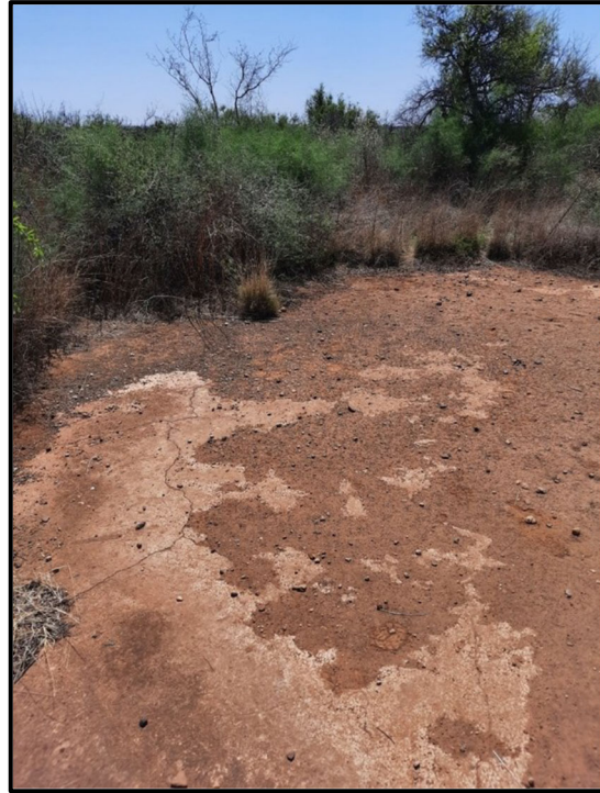
Figure 8.7. Cement floor at FEAT 02
