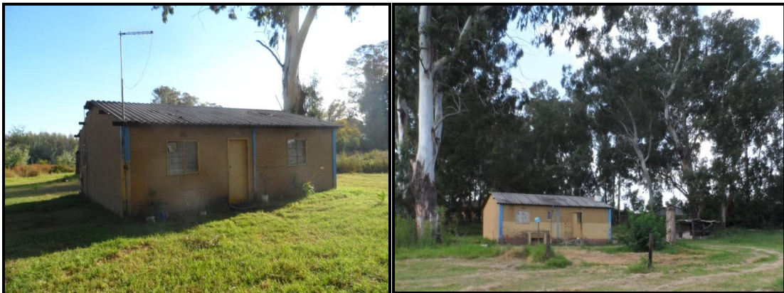
Figure 10- Structure with asbestos roof (1960s).
