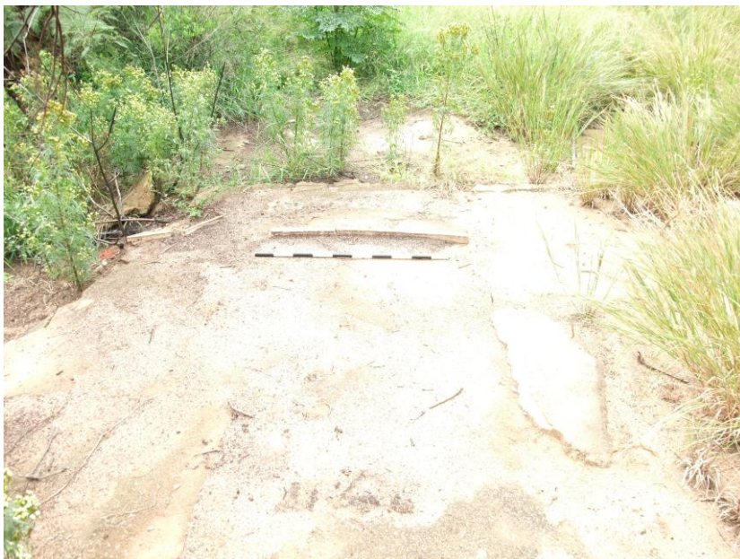
FIGURE 17: REMAINS OF ONE OF THE CONCRETE FLOORS.
