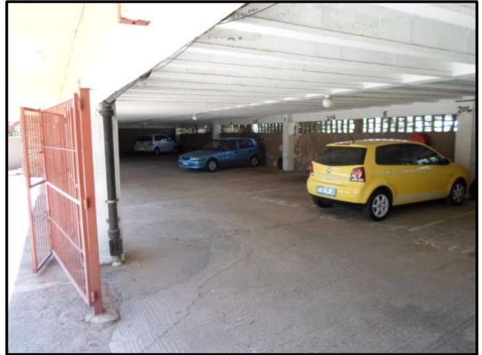
Figure 15. Underground parking area.
