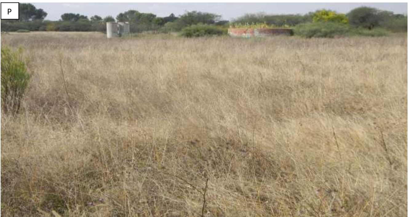
Plate 16: Photo P. showing delapidated water reservoir within the proposed township establishment site.
