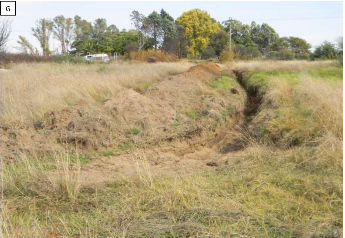
Plate 6: Photo G. showing a sewer trench within the proposed township establishment site
