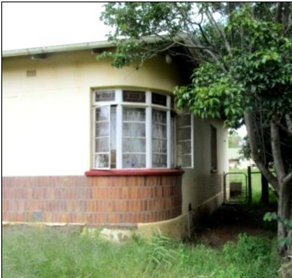
Figure 7. Arced "corner" window – note four panes.
