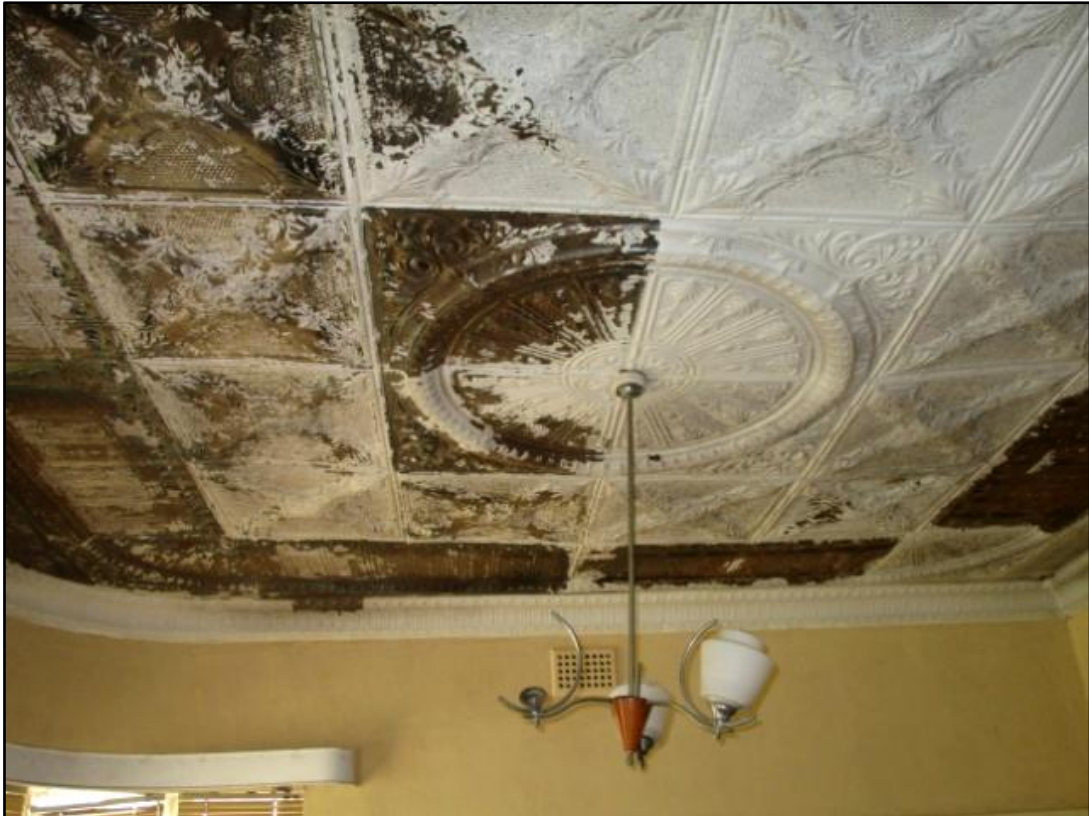
Figure 16. Pressed metal ceiling with scraped off paint.
