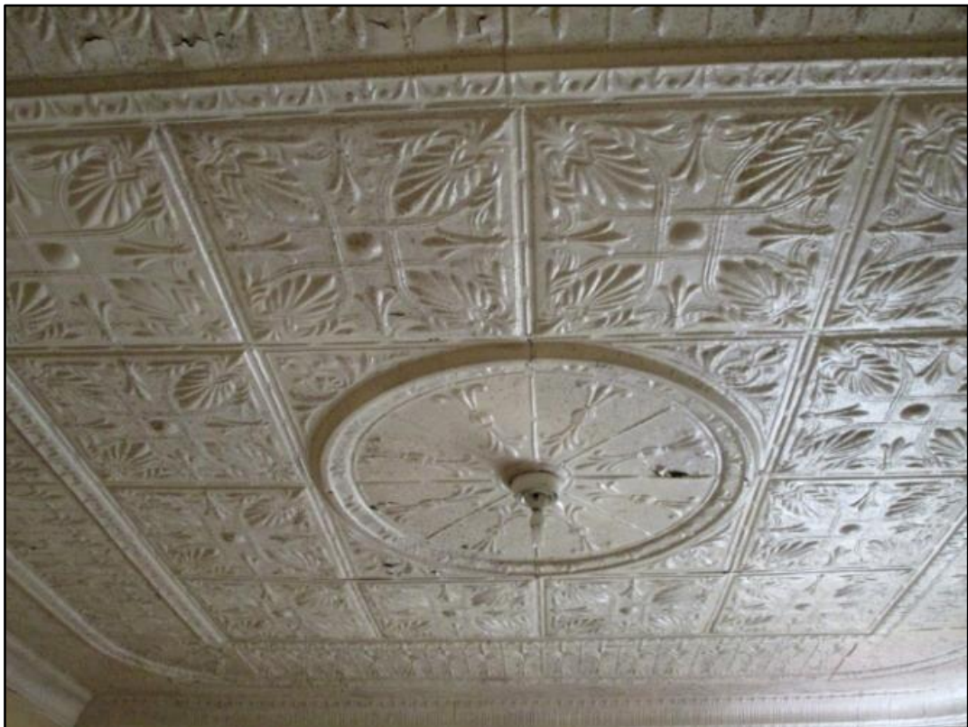
Figure 15. Pressed metal ceiling.
