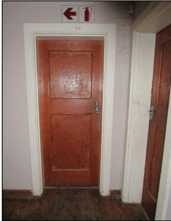
Figure 6. Solid panelled doors in the house.
