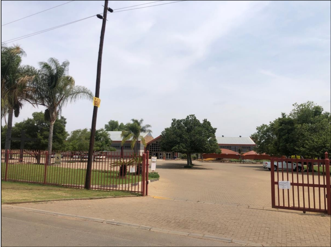
Figure 12. Entrance to the existing church on the Remainder of Portion 220 of the Farm Sterkloop 688-LS
