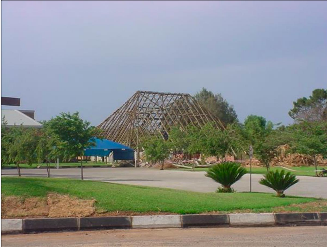
Figure 14. View of the existing church on the Remainder of Portion 220 of the Farm Sterkloop 688-LS
