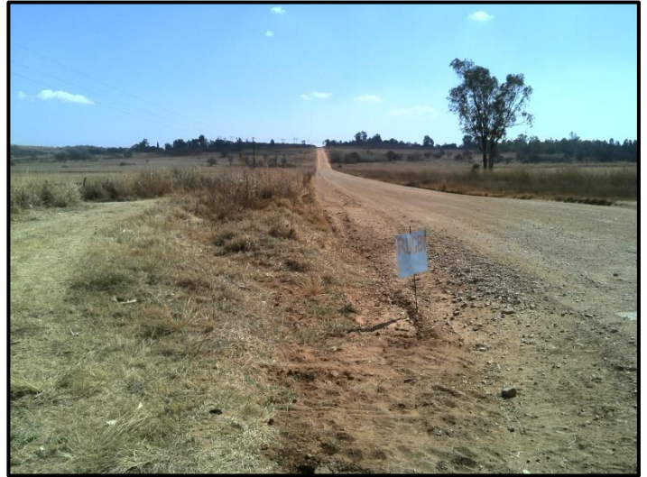
Figure 5. General site conditions
