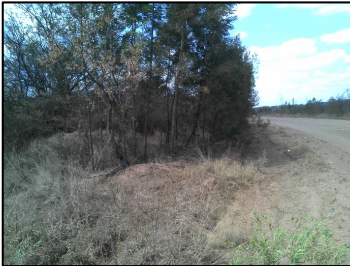
Figure 6. Overgrown section of the road reserve.
