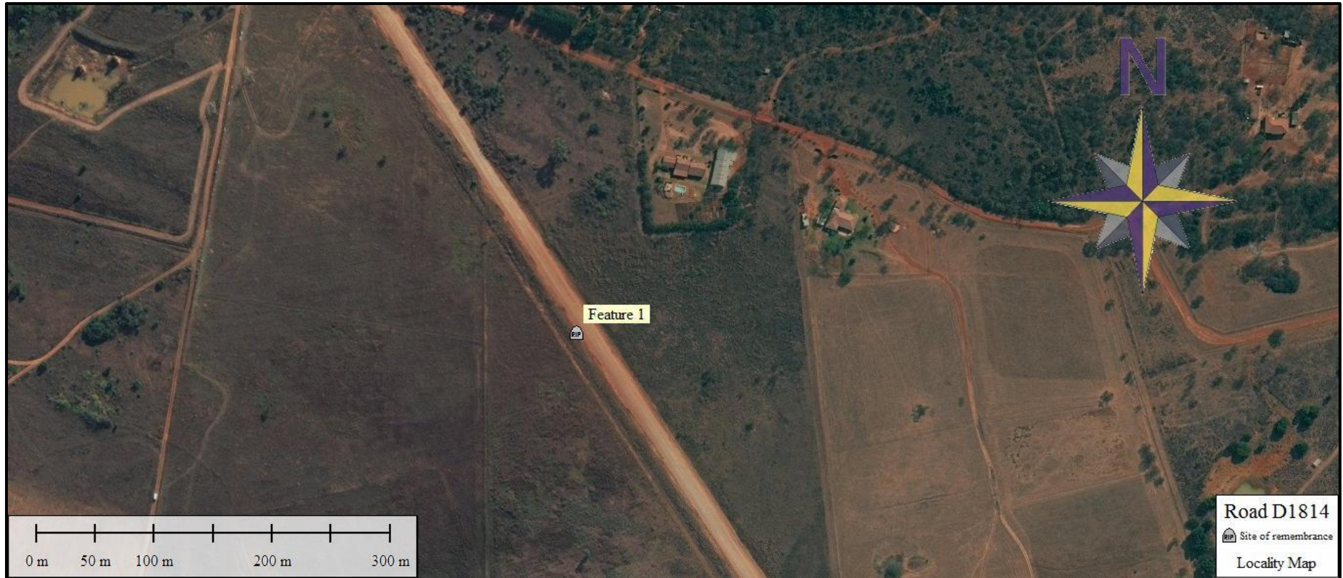
Figure 16: Location of Feature 1 within the road reserve.
