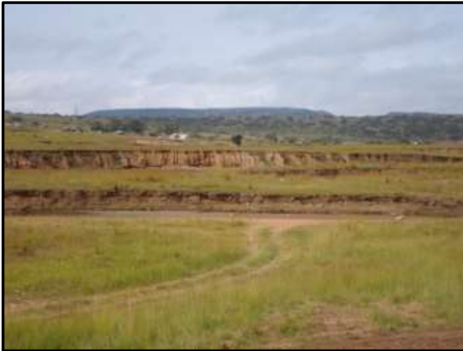
Figure 7. Erosion in the southern portion of the study area.
