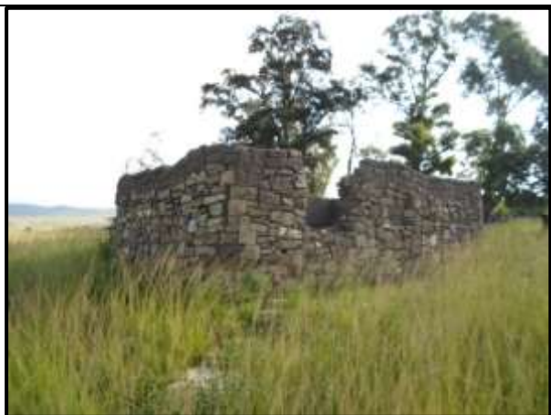
Figure 22. Stone built structure at R5.
