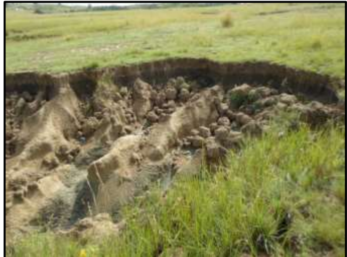
Figure 8. Erosion in the southern portion of the study area.
