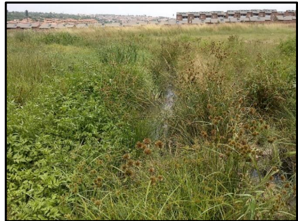
Figure 7-4. Sewage flowing through the study area.
