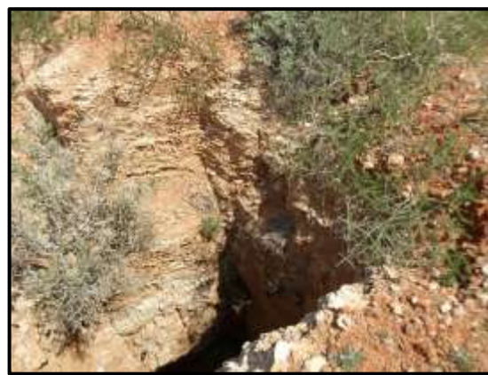
Figure 18. Excavation through calcrete substrata.
