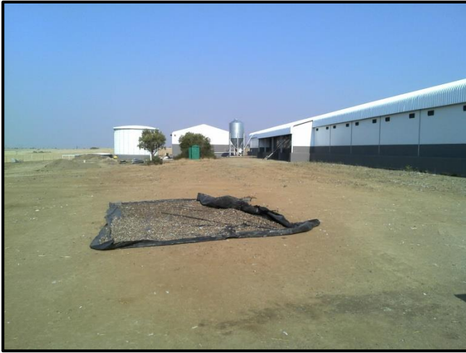
Figure 5. General site conditions – Alternative 1.
