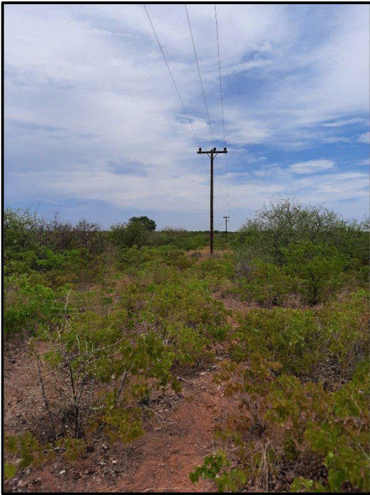
Figure 7.1. Existing Powerline infrastructure viewed from Option 1.
