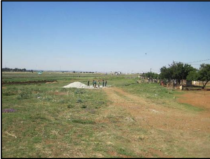
Figure 5. General site conditions
