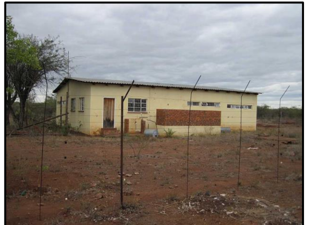
Figure 20. Buildings in the study area
