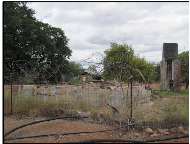
Figure 18. Buildings in the study area
