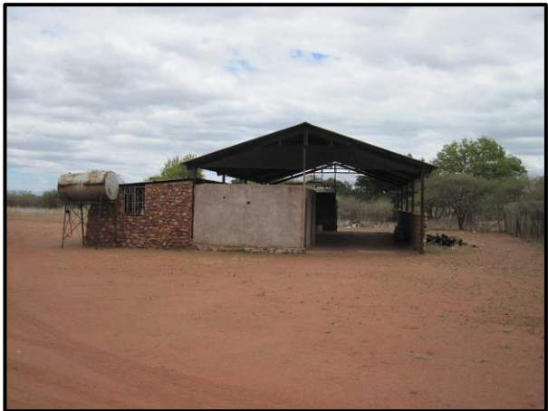
Figure 19. Structures in the study area.
