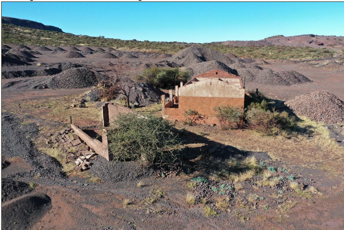
Figure 33. Crusher dumps and abandoned infrastructure
