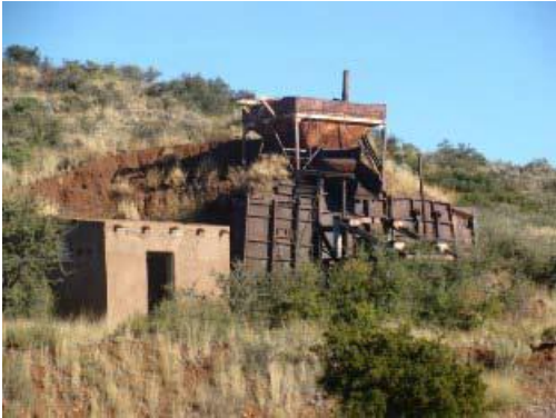
Figure 15. Ore crushing plant
