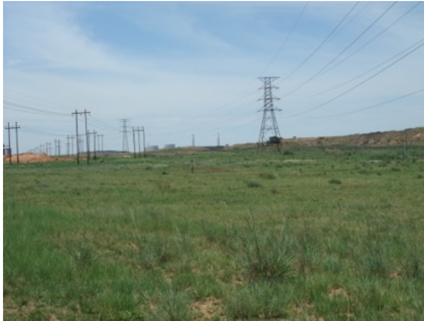
Figure 6: View of vegetation along the existing line. Note the mine dumps on both sides.
