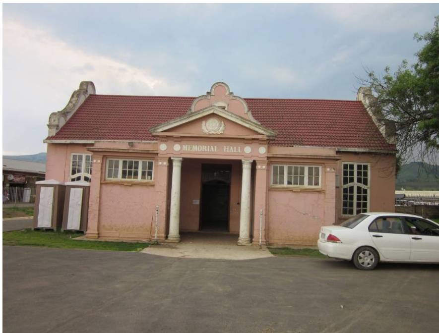
Fig 1: Front elevation of building
