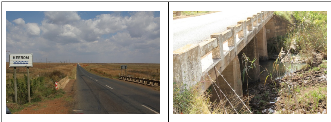
Fig. 8. Views of the Keeromspruit bridge.
