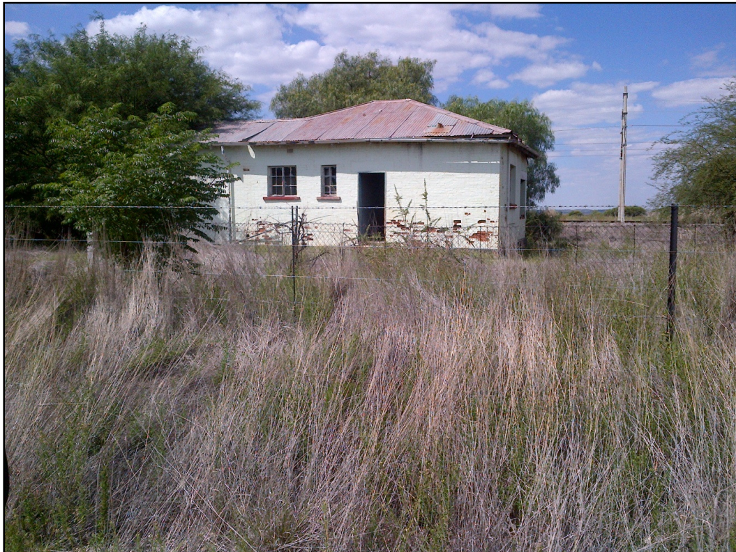
Figure 7: Historical structures are located west from the existing railway line at Heuningneskloof, but they will not be impacted by the proposed borrow pit development
