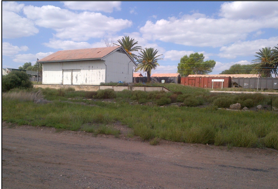
Figure 12: Old railway structures are located at Belmont station, but they will not be impacted by the proposed borrow pit development
