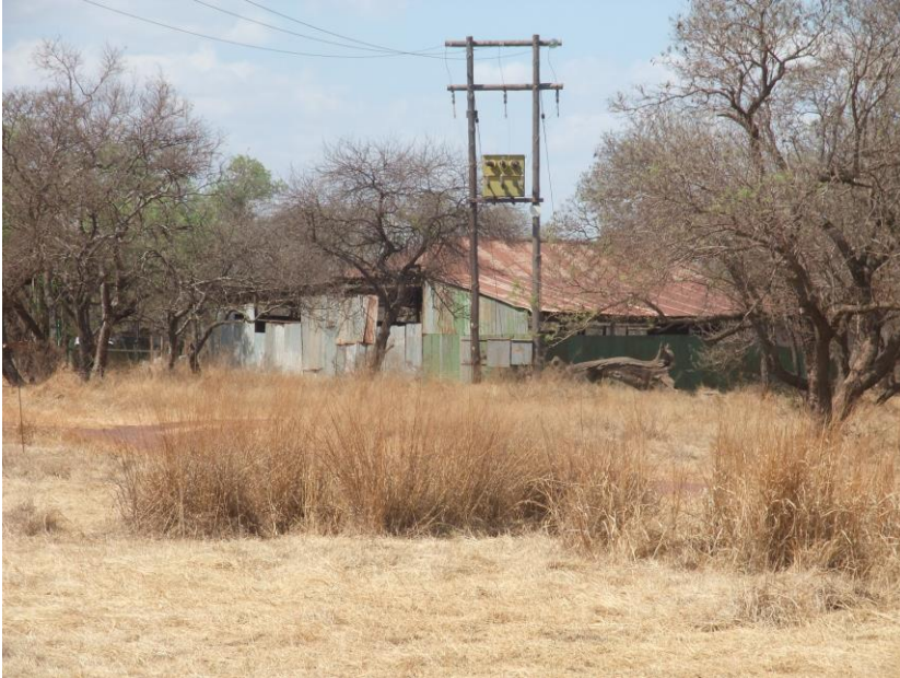
Figure 6: General view of the area where the substation for Alternative 2 is planned. The corrugated iron building falls outside of this area, but has no heritage significance and is currently used as a workshop.
