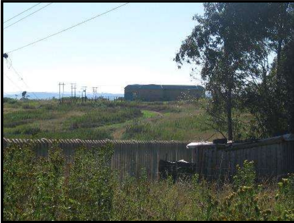
Figure 5. Start of the proposed preferred route near the new pump station to the east of Midmar Dam. No heritage sites occur in this area.
