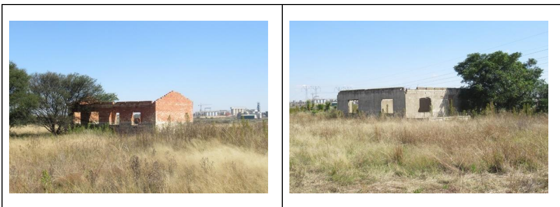
Figure 14. Abandoned, recent structures on the western section of the project area
