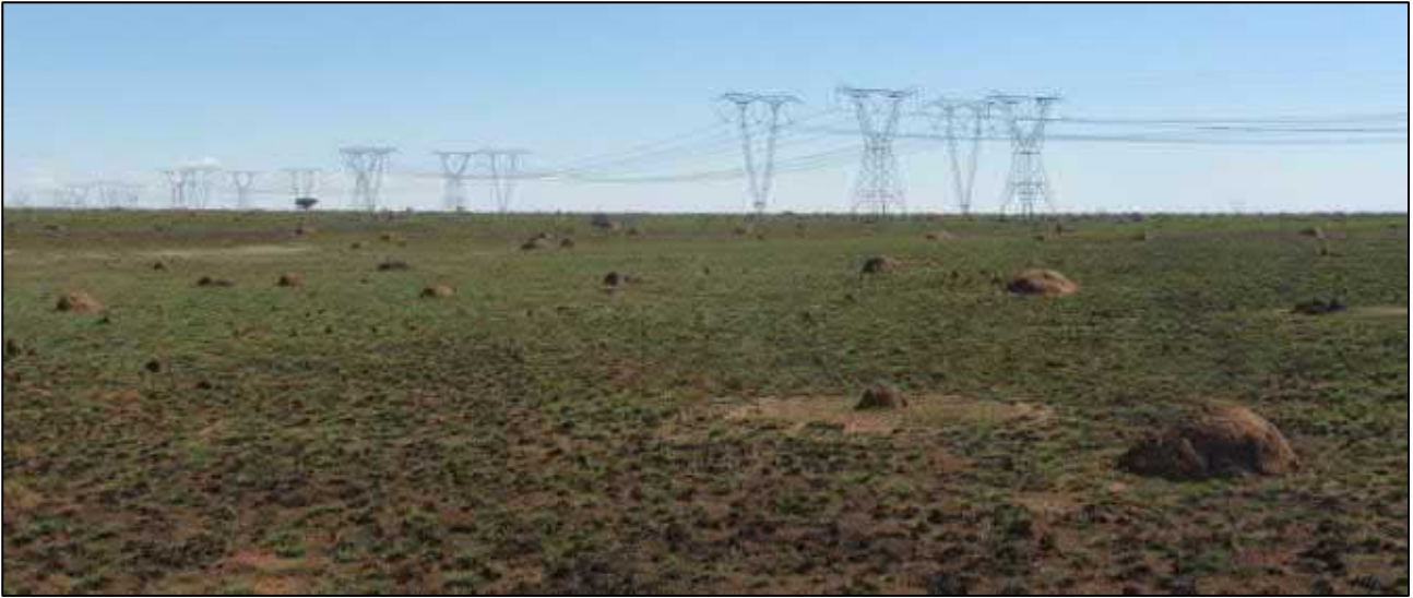
Figure 13: View towards the southwest from the point where the proposed powerline corridor crosses the R64.
