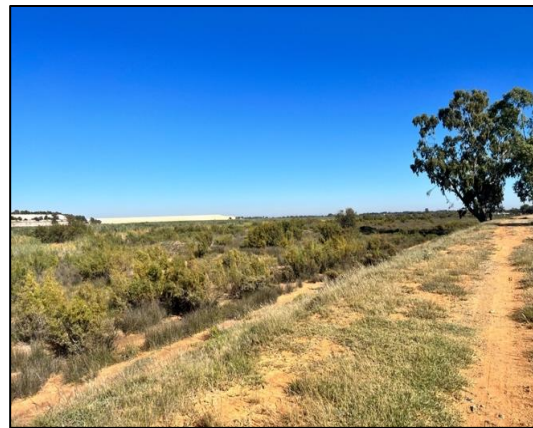
Figure 19 – View of the area near Dam 13.
