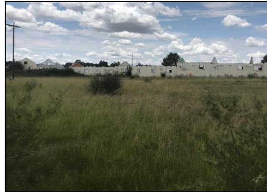
Figure 15 – View of disused residential compound.
