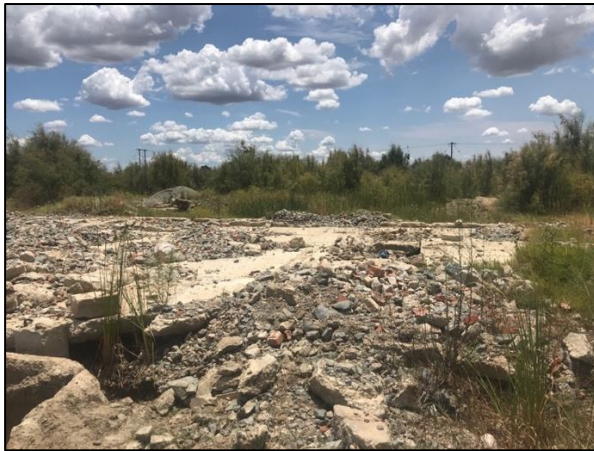
Figure 12 – View of demolished structures.
