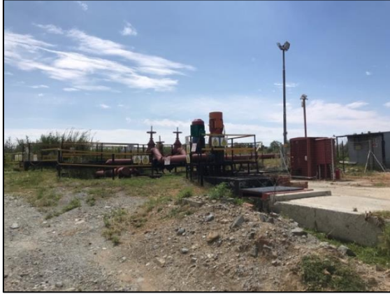
Figure 10 – View of existing pipeline infrastructure.
