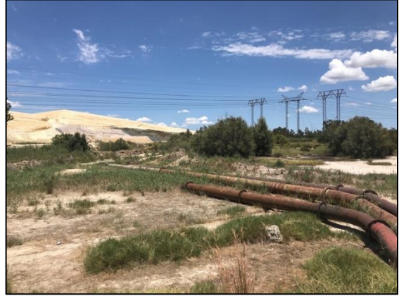
Figure 11 – View of existing pipelines.
