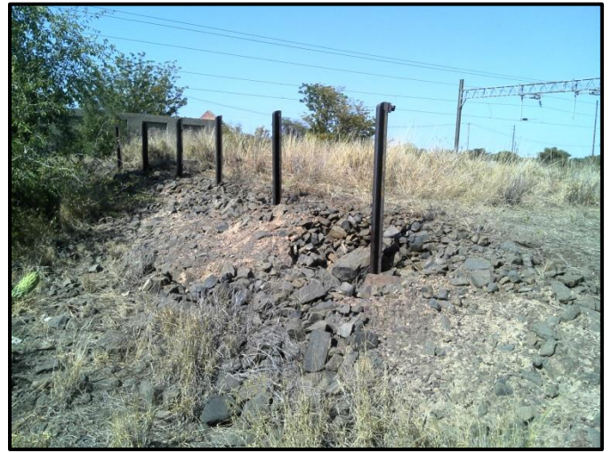
Figure 21. Remains of loading ramp at Site 4b.
