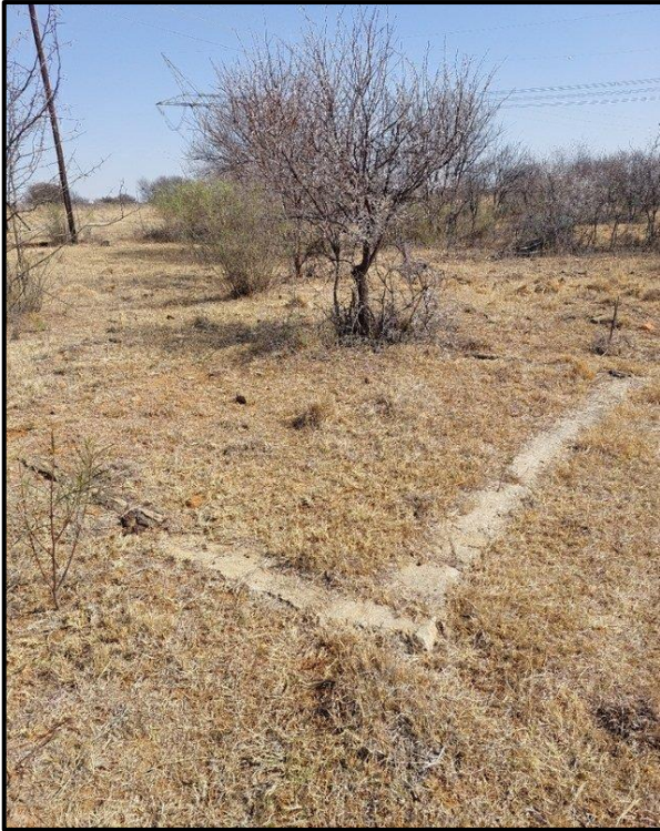
Figure 7.28. Ephemeral cement foundation at BV009 – The feature is totally demolished.
