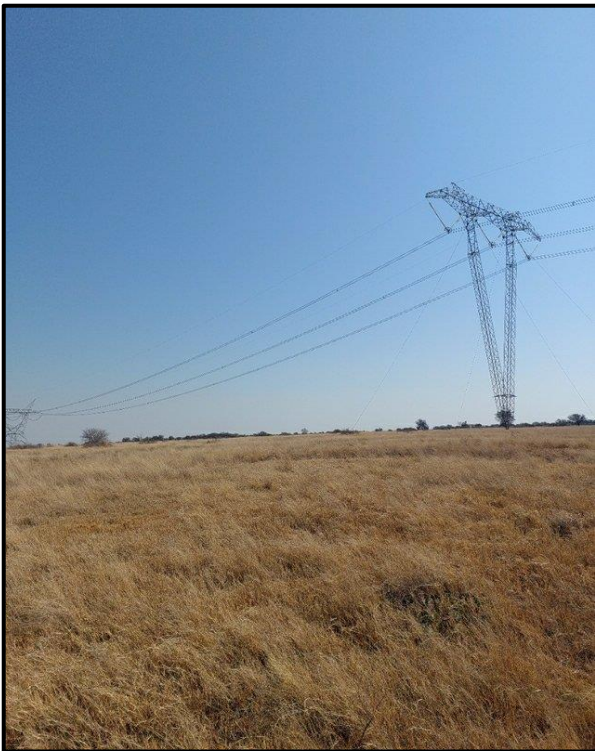
Figure 7.3. Image showing the existing powerlines across the north western corner of the Project area.
