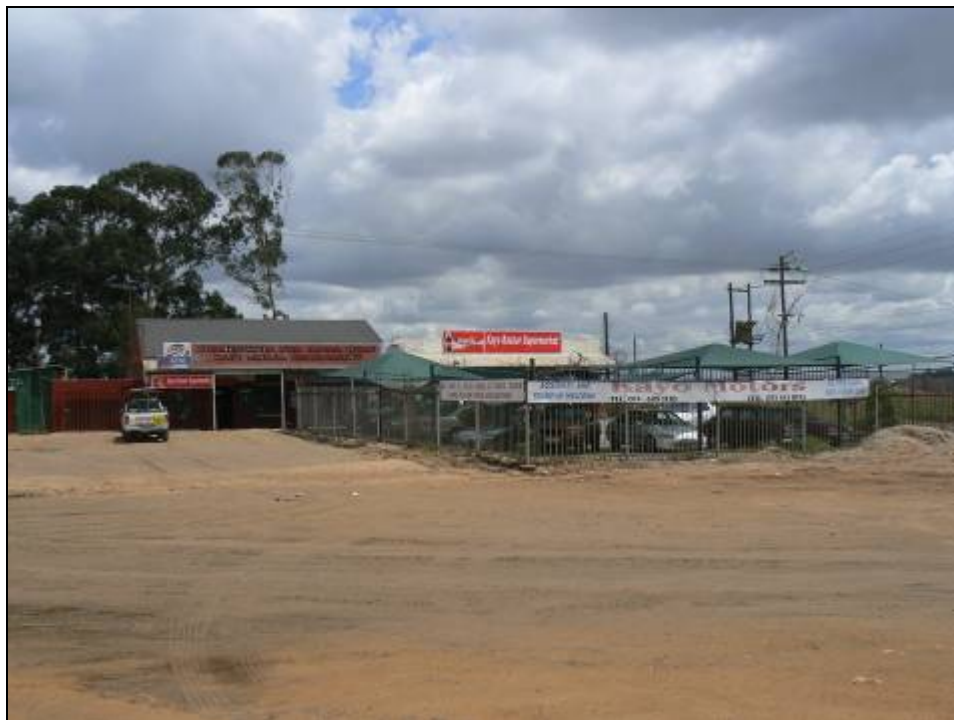
FIGURE 16: Kayo Bazaar (S 1). This building is probably older than 60 years but will not be affected.
