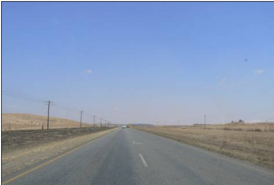
FIGURE 10: Section of Road R 547 south of Ga-Nala (Kriel) where the pipeline (E-F) will run next to the road
