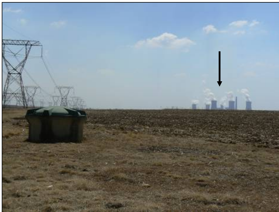
FIGURE 11: Air vent of the existing DWAF pipeline between Matla (arrow) and the Rietfontein Pumping Station, amended route section A-B-C-D
