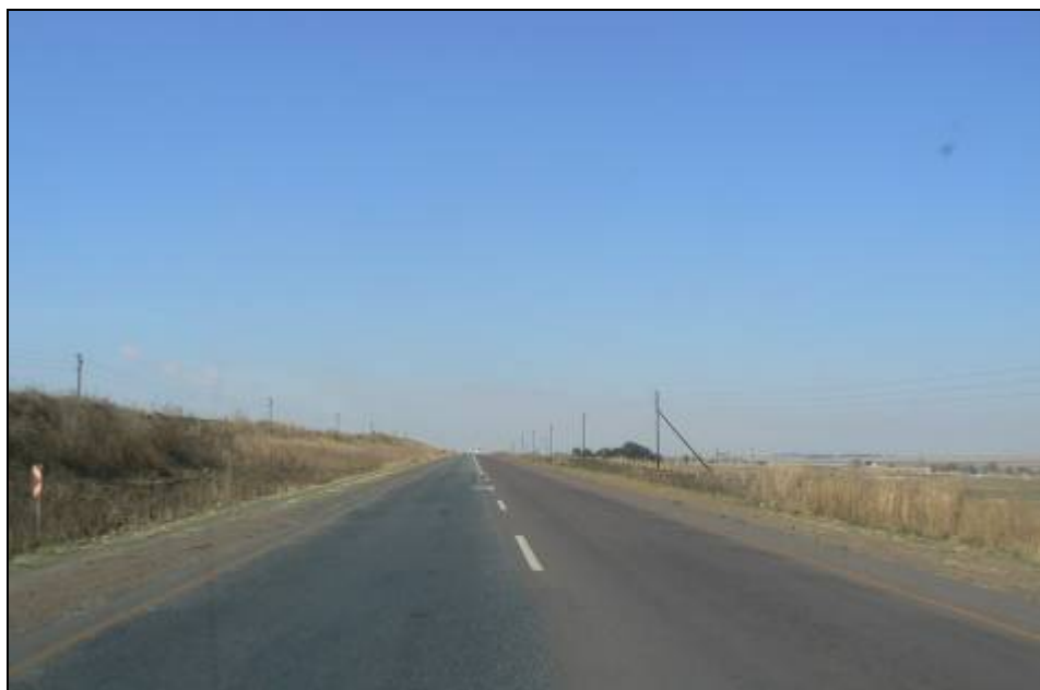
FIGURE 8: Section of Road R 544 between Duvha and Van Dyksdrif (G-H) where the pipeline will run next to the road
