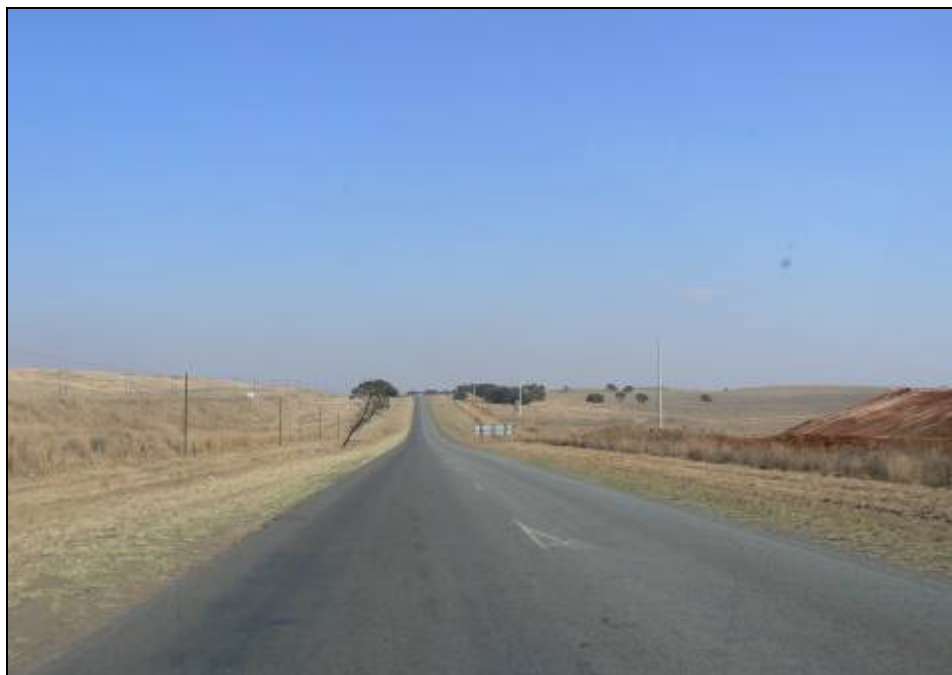
FIGURE 7: Section of Road R 575 south of Duvha where the pipeline (authorised and amended routes I-H) will run next to the road
