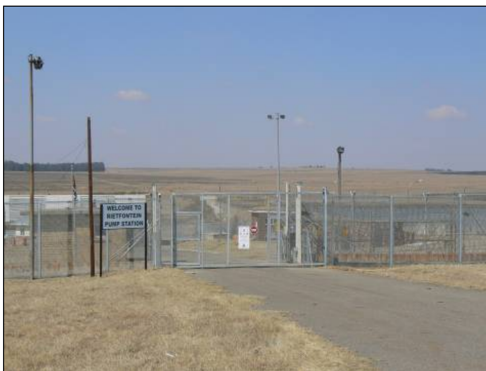
FIGURE 12: Rietfontein Pumping Station
