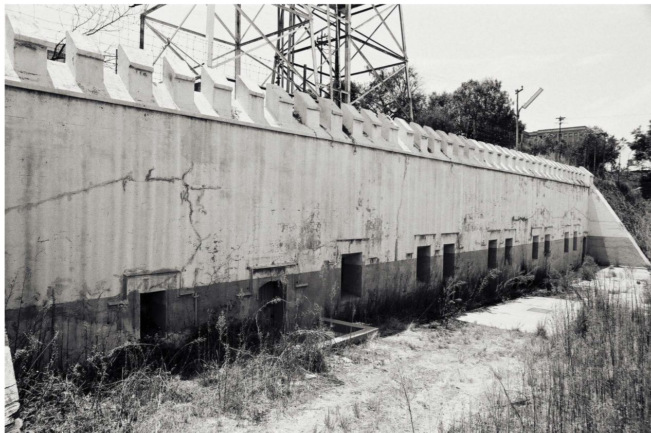
Figure 22: The eastern rampart rooms and water tower circa 1985 after the closure of the prison (Chris Reilly via Herbert Prins)
