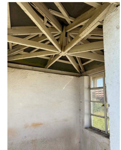
Figure 41: North east guard house interior
