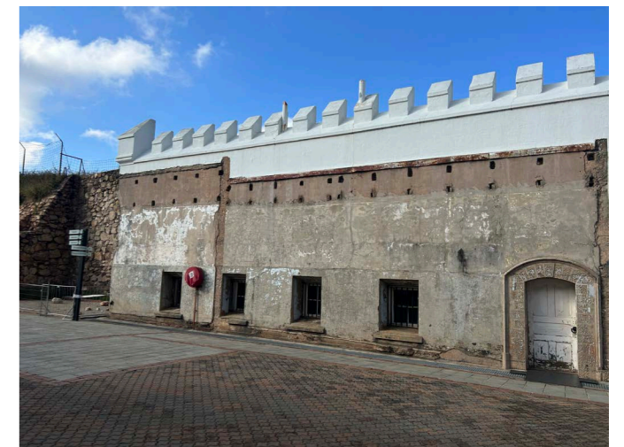
Figure 12: Demolished reception rooms
