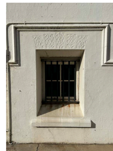
Figure 11: Southern rampart window
