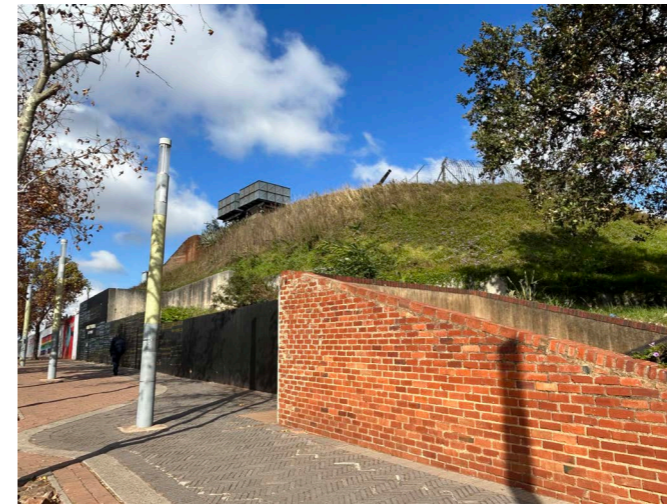
Figure 48: Exterior view of western rampart
