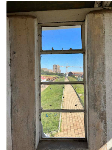
Figure 38: North east guard house window
