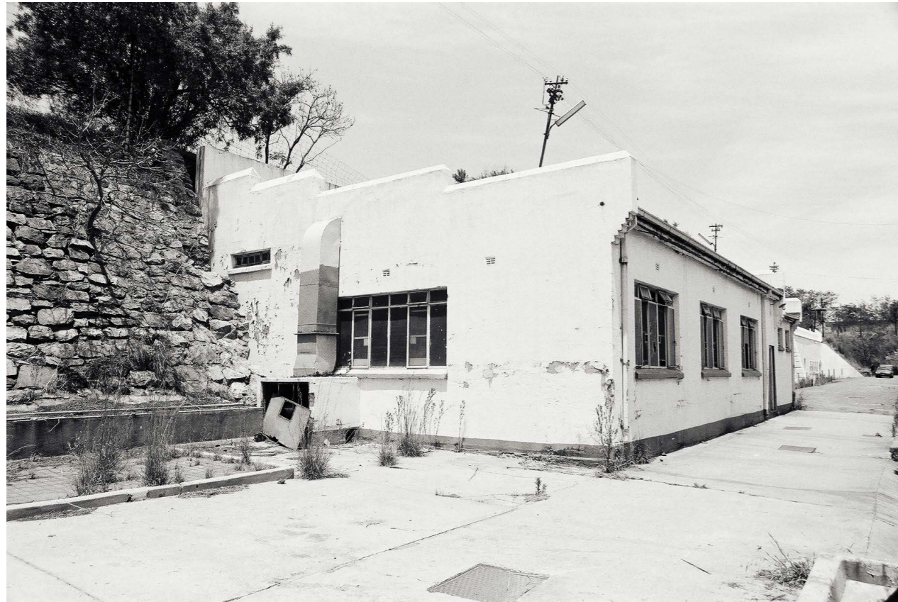
Figure 21: The now demolished reception rooms in front of the retaining wall that is proposed to be rebuilt circa 1985 after the closure of the prison (Chris Reilly via Herbert Prins)
