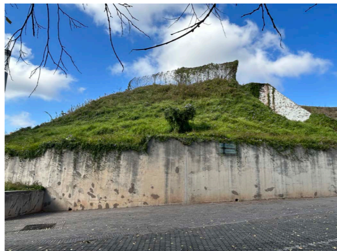
Figure 47: Exterior view of northern rampart
