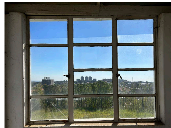
Figure 40: North east guard house window
