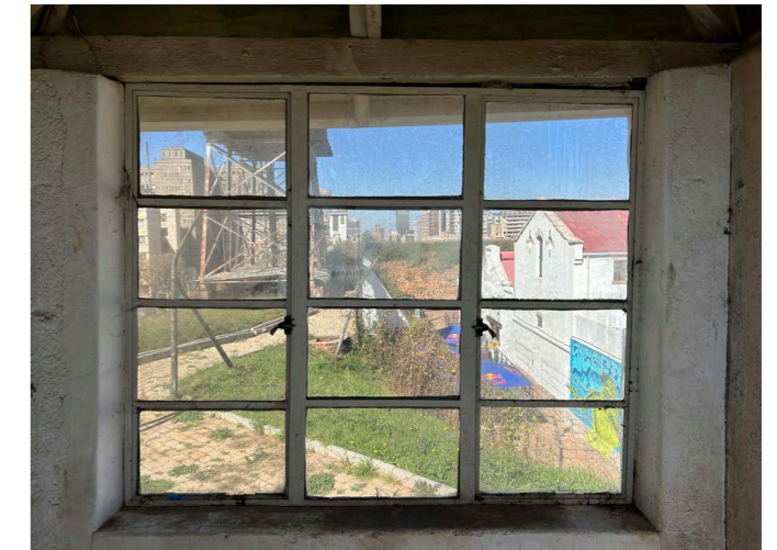
Figure 39: North east guard house window
