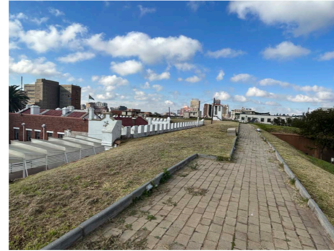
Figure 18: Path on western rampart toward the south
