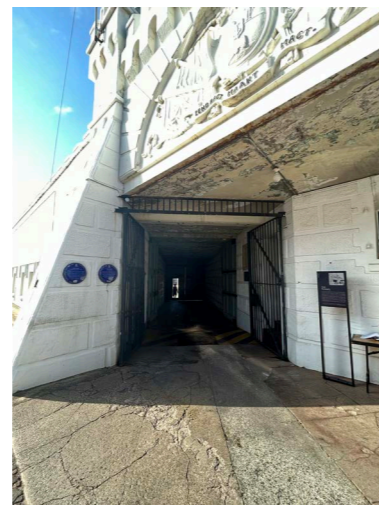
Figure 6: Tunnel under rampart
