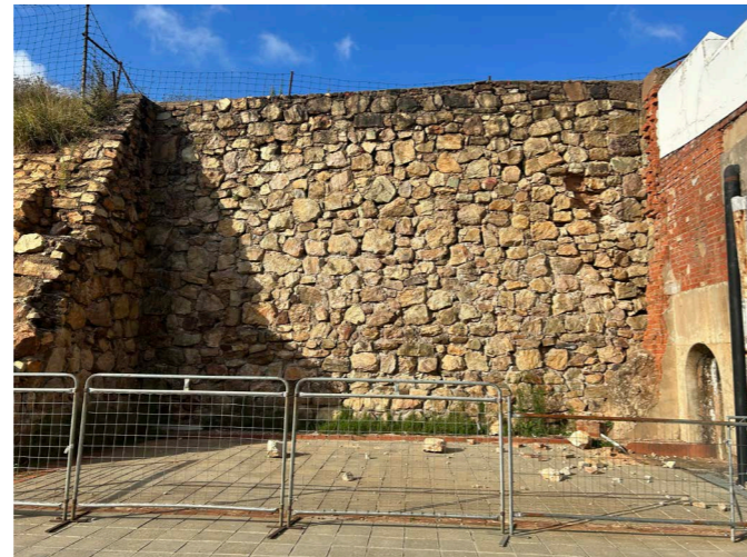
Figure 16: Vertical retaining wall on southern rampart
