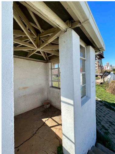
Figure 42: North east guard house entrance
