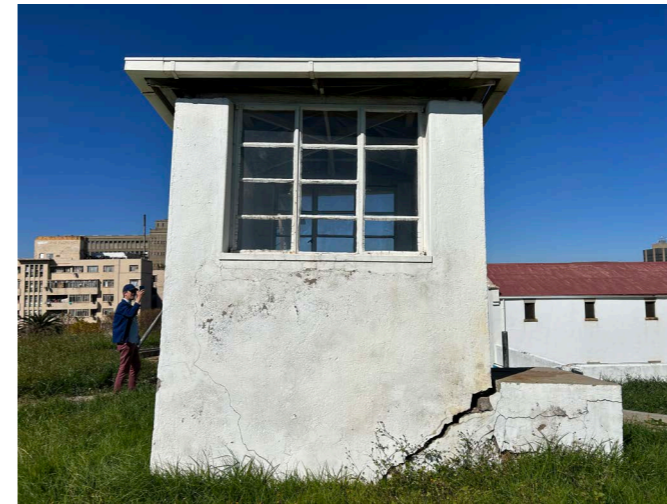
Figure 36: North east guard house northern facade
