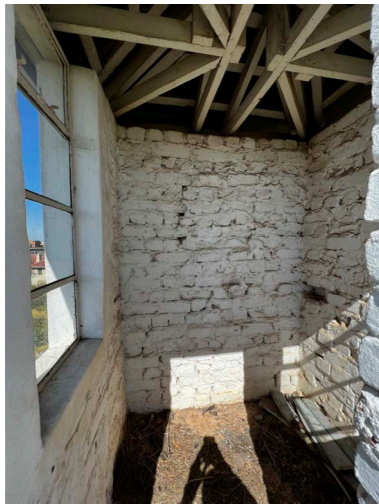
Figure 18: Interior of south west guard house
