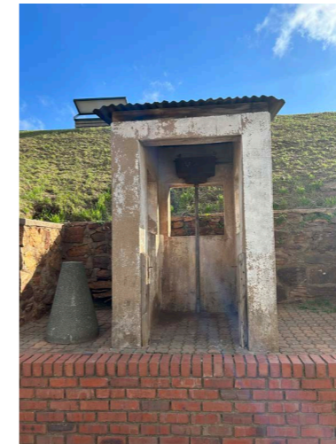
Figure 21: Guard house at base of southern rampart
