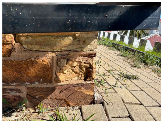
Figure 22: Vent shaft stone wall
