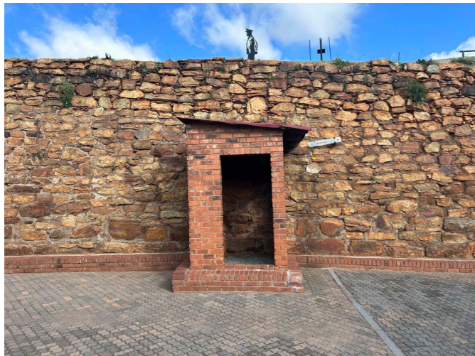
Figure 44: Face brick guard house
