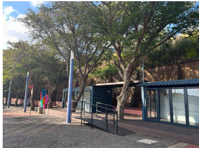
Figure 45: Exterior view of northern rampart
