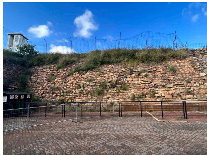
Figure 17: Inclined retaining wall on southern rampart
