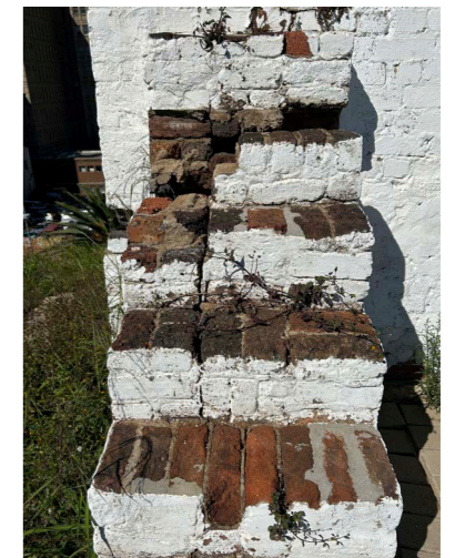
Figure 27: South east guard house brick steps
