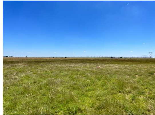
Figure 7 – General view of Good Hope substation area at the north eastern end of the GHOHPL proposed corridor
