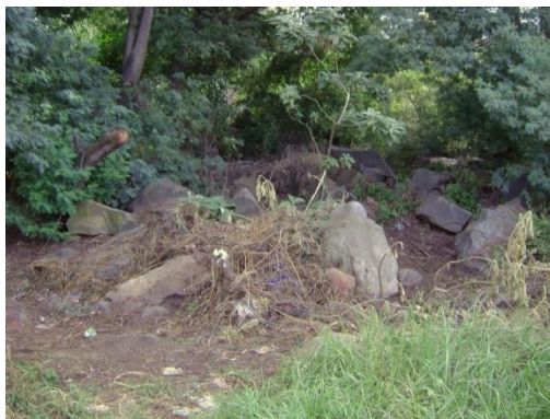
Downstream side of the dam wall
