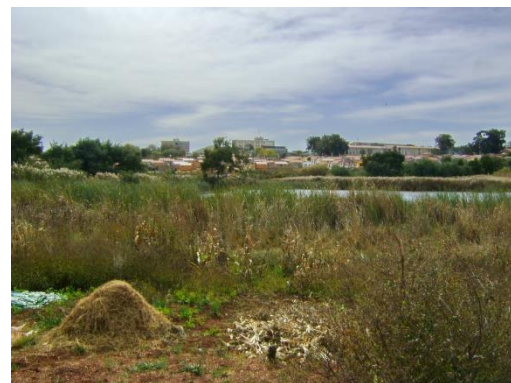
View across the dam looking north
