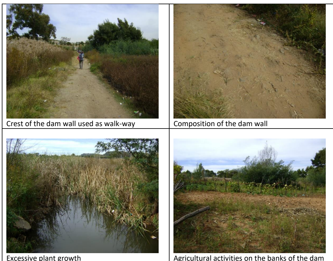
Figure 8. Various elements regarding the dam
