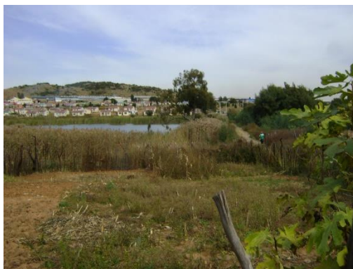
View across the dam looking south
